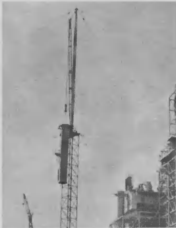
One major lift is handled by the 307-ft. derrick crane: a section of the PCAR smokestack. In about half an hour of skilled maneuvers, upward and downward, the section came down safely on the ground.
